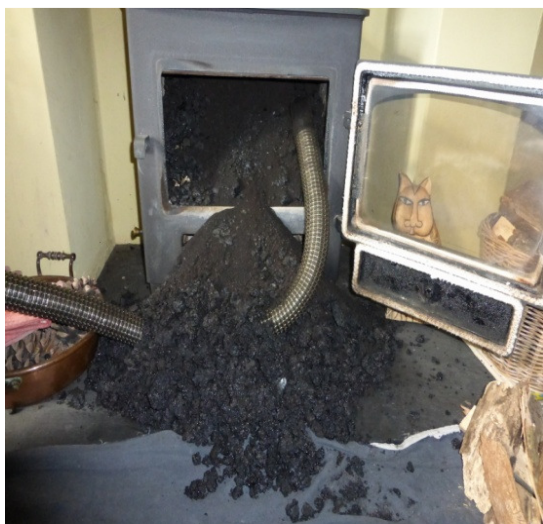
Good stove, dry wood, good chimney but the air was closed off too much
